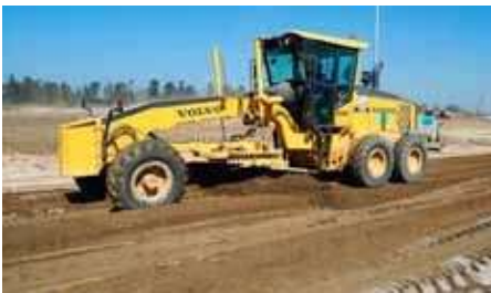
Levelling with a Grader
