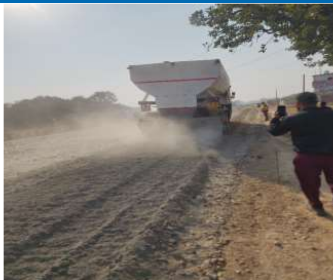
Milling/ pulverization
