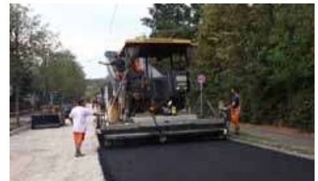
Installation of asphalt after 48h
