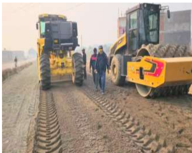
Grading and Rolling
